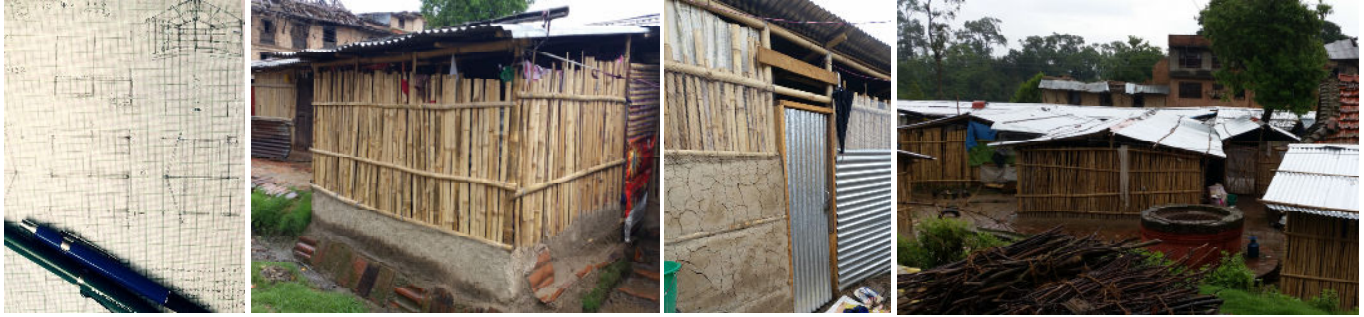
Figure 8 Shelters built by KU Center for Art & Design Faculty and students in the village of Bungamati after the devastating earthquake in April 2015
